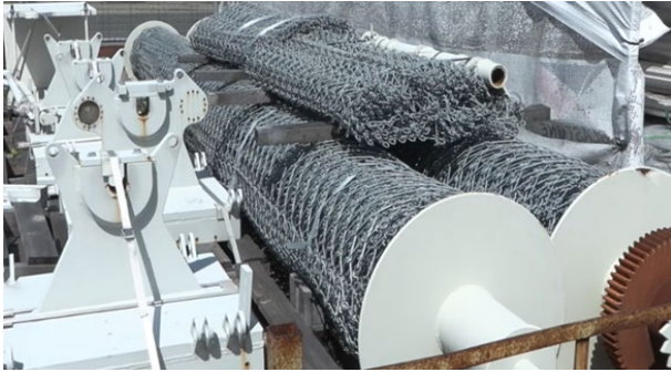
Figure 8 Snapback arresting structure components ready for installation at the lay down area at Hay Point - Poulter B, (2025)
