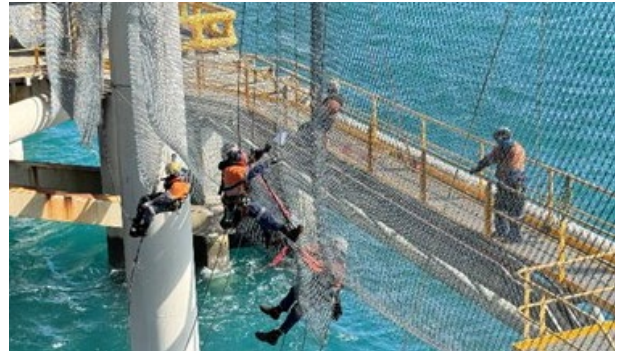
Figure 10 Rope access team during installation of the snapback arresting structure – BMA, (2024)
