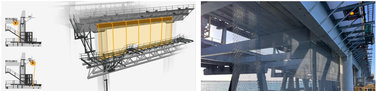
Figure 1 Snapback roller deployment system concept - Vollebregt J, (2023); Hay Point Coal Terminal under-berth work zone - BMA (2025)
