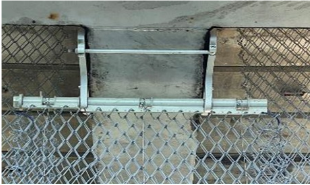
Figure 17 Traversing support beams were accommodated using saddle bracketry and infill panels – BMA, (2024)
