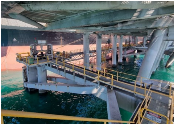
Figure 3 A typical under berth area at BMA Hay Point where the pile refurbishment work is required – Keane R, (2023)
